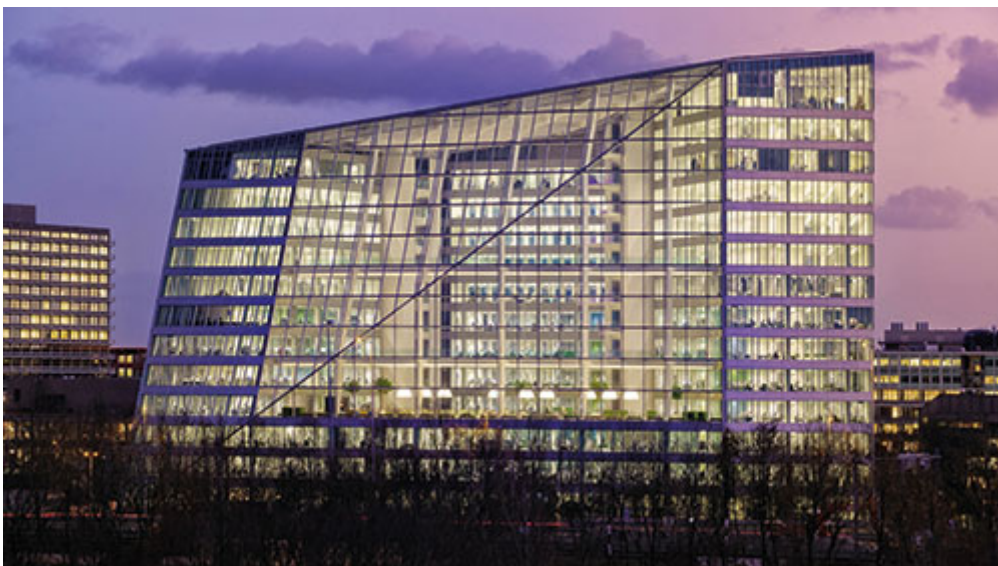
The Edge in Amsterdam is one of the world's most high-tech offices (Credit: Ronald Tilleman)
